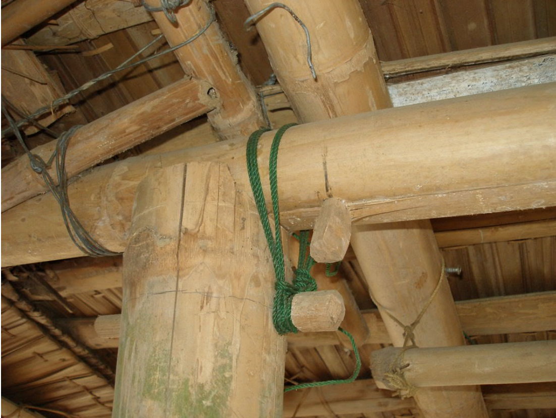
Bamboo supports, joints, & beams in a structure in the Philippines
