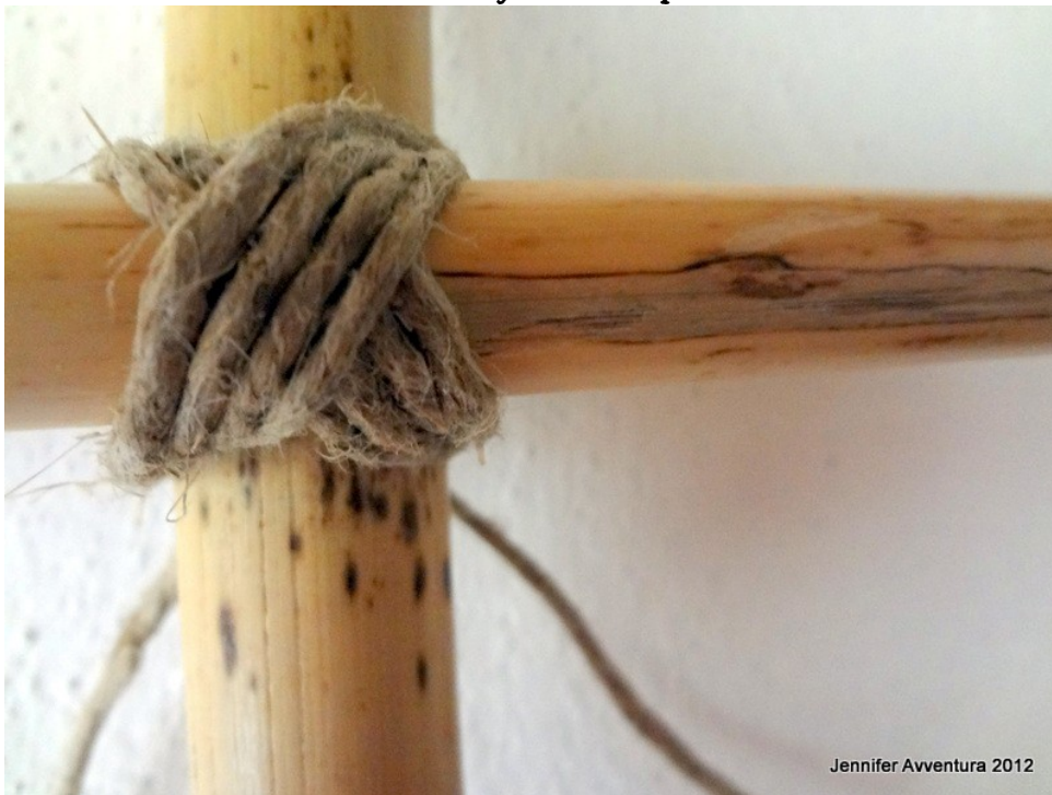
Bamboo ladder, cut to fit on each piece then lashed
