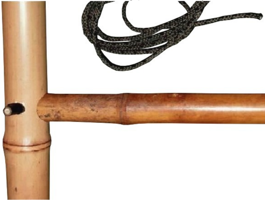
Bamboo ladder, joined with peg & later lashed for stability
