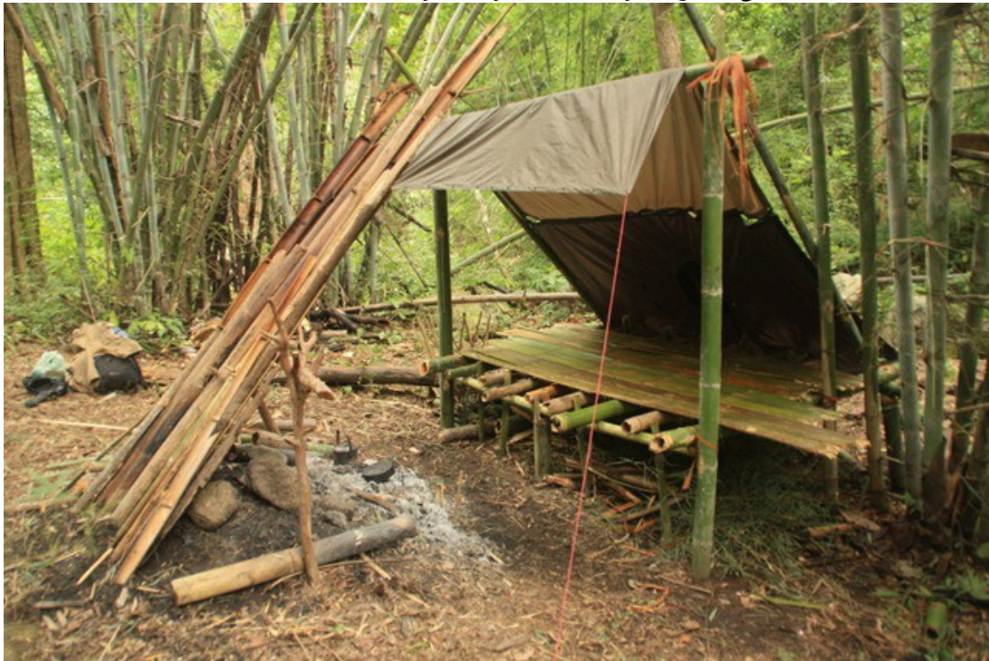
Bamboo shelter with fire reflector and flat plank floors
